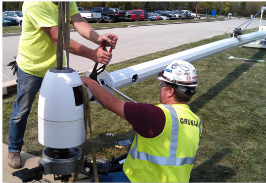
Installing the turbine head on the tower
