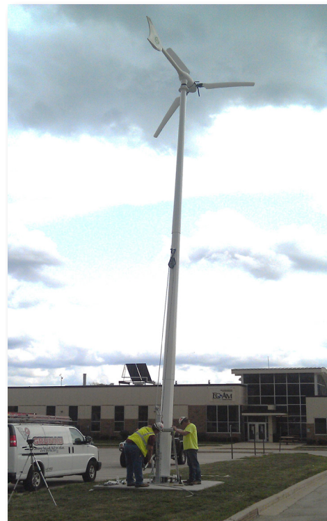
Raising the wind turbine
